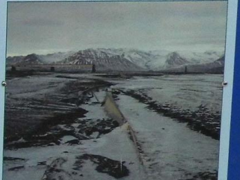
Mynd: Vaggarðinn The damage caused was very evident when the flood was over and it was clear that there was costly rebuilding ahead. The picture shows a steel beam from the bridge over Skeiðar half buried in mud far down the river. Skemmdir komu því vel í ljós þegar hlaupin lauk og auglöst var að víðgerðarstærð yfir Gígukvísl. Eftir hlaupin lagu stálar frá Skeiðarbrúni halgrunnir í frambrúnaður langt niðan brúna.
