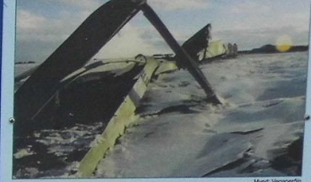
Mynd: Vaggarðinn Eyðilegging / Destruction Mikil fjöldi þaka barist með Hlaupavötnu nór á sandinn og alla löd í sig fram. Áætlað er að þakarnir sem náðu nór á brúarstæðinu við Gígukvísl hafi veði afir að 1.000-2.000 tonn (samsvartar í umlíti þrogga hafa þarhúsi) en að þakarnir sem náðu nór á brúna yfir Skeiðar hafi veði afir að 100-200 tonn. Skemmdir af vöðum þakna voru gráðarmiklar. Many large blocks of ice were carried across the sandflats by the flood, some even out to sea. Those that were carried as far as the site of the bridge across the Gígukvísl are estimated to have weighed as much as 1,000-2,000 tons, while the ones that reached the bridge over the river Skeiðar were up to 100-200 tons. The caused immense destruction, when the floodwaters receded it was clear that road repairs would be very expensive. Steel girders from the Skeiðar bridge were left half buried in sand far downstream from the bridge after the flood.
